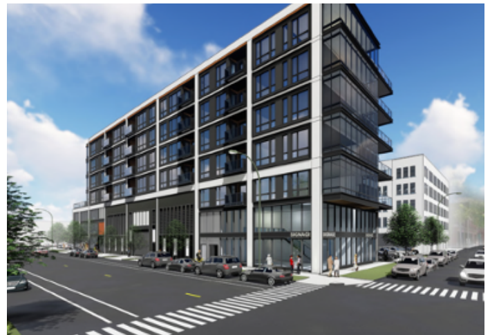
Rendering of multi-use development that surrounds Juneautown substation Photo: Rinka Chung / Joseph Property Development
