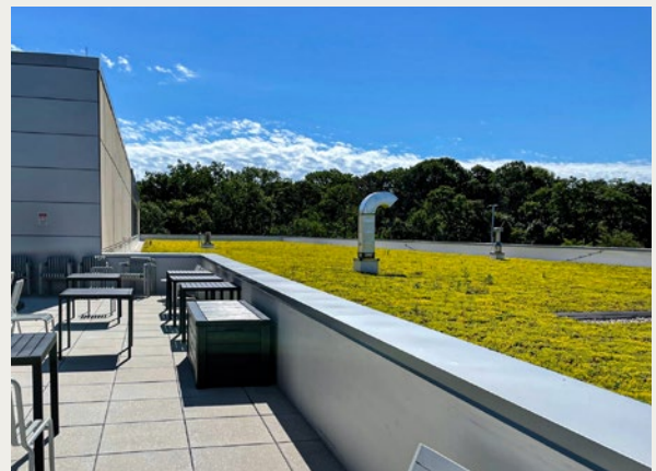
View of the green roof at the Peoples Gas North Shop
