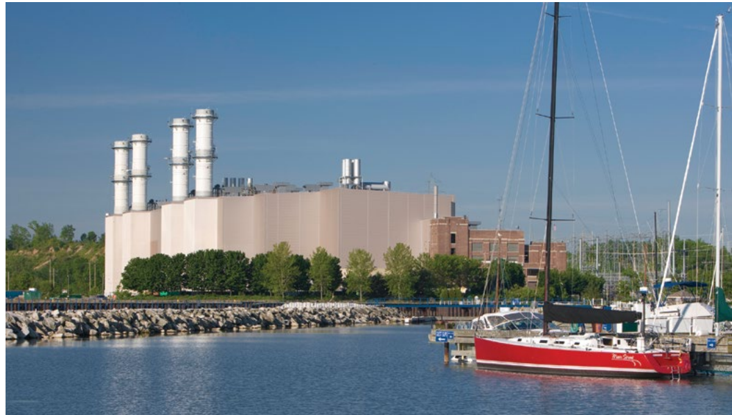
Port Washington Generating Station
