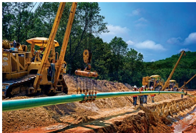
West Central Gas Expansion
