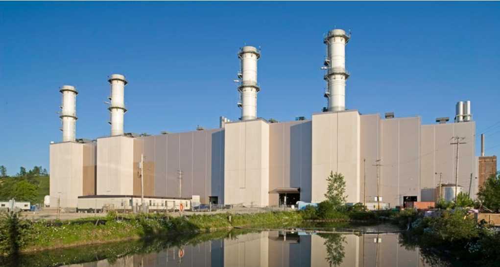
Port Washington Generating Station
