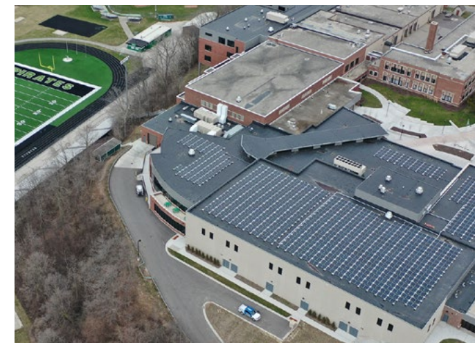
A Solar Now array at a Port Washington school
